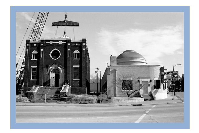
We've had cranes at the Synagogue all month, replacing the roof and the HVAC units on top of it. The equipment lasted just under twenty years, a ripe old age for this kind of machinery.
